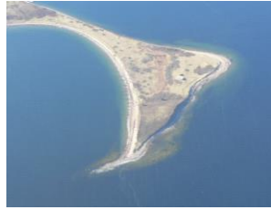
Masons I Northern end
